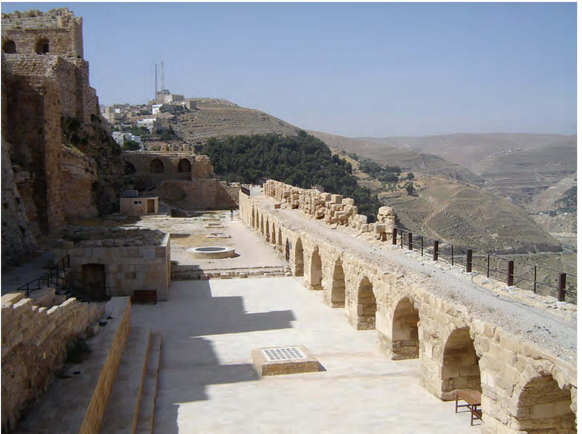
Kerak, line of casemates built by the Mamlūks along the outer western wall. (Michael Fulton)
